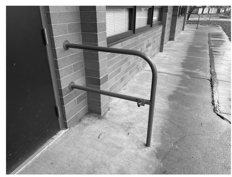
**EXISTING CONDITIONS, PIPE RAILING** - MATCH CONSTRUCTION FOR NEW DOOR STOP - 1 1/2" STEEL PIPE ASSUMED, 36" LONG, FIELD
