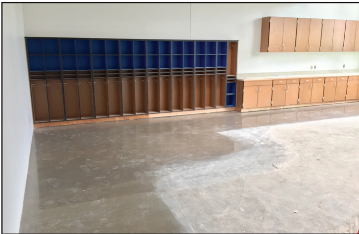
Concrete polishing and casework
