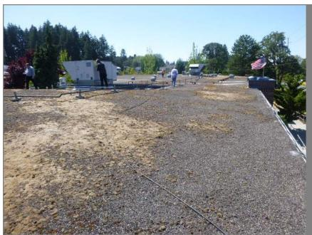
Overview of main roof (Roof Area 'A') as viewed from NE corner looking west. Photo taken before moss removed for the moisture survey.
