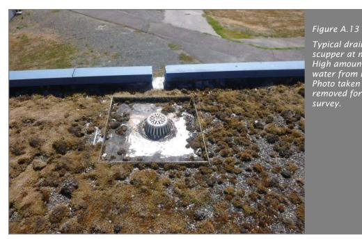
Typical drain and overflow scupper at modular building. High amount of moss prevents water from reaching drain. Photo taken before moss removed for the moisture survey.
