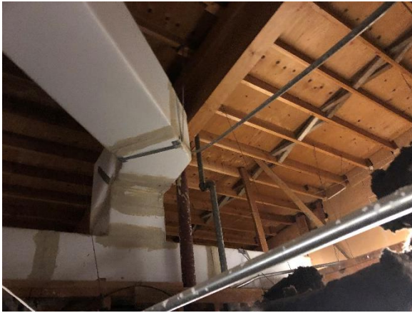
Figure 13: Unblocked plywood roof diaphragm
