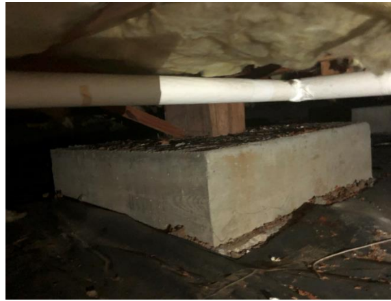
Figure 14: Absence of blocking for load path transfer
