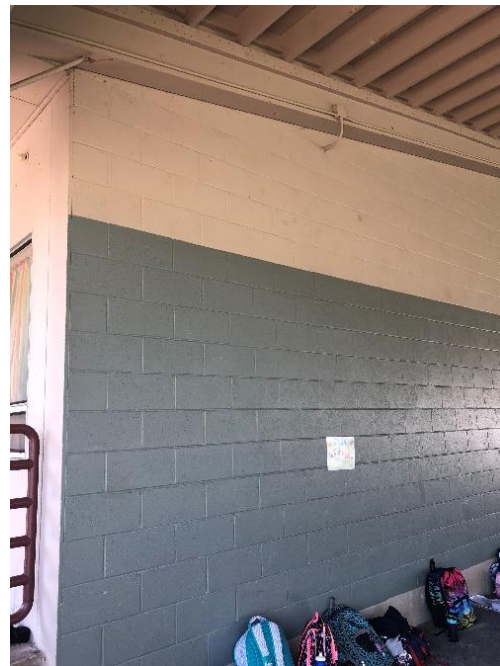
Figure 12: CMU wall at covered play area of Building Part C2
