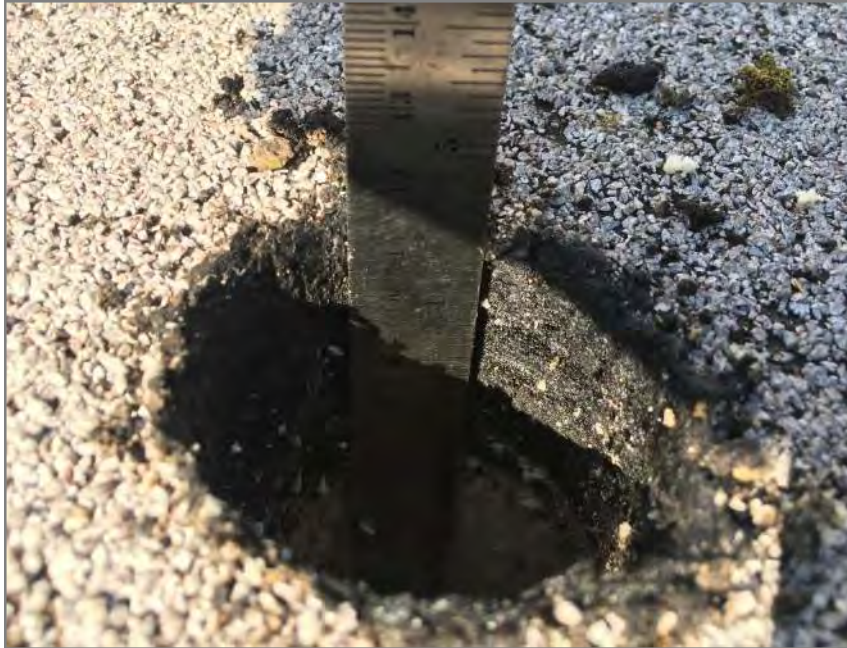
Figure C.11 1/2" walk pad 1" BUR 1/2" fiberboard 2-1/2" polyiso insulation Concrete deck
