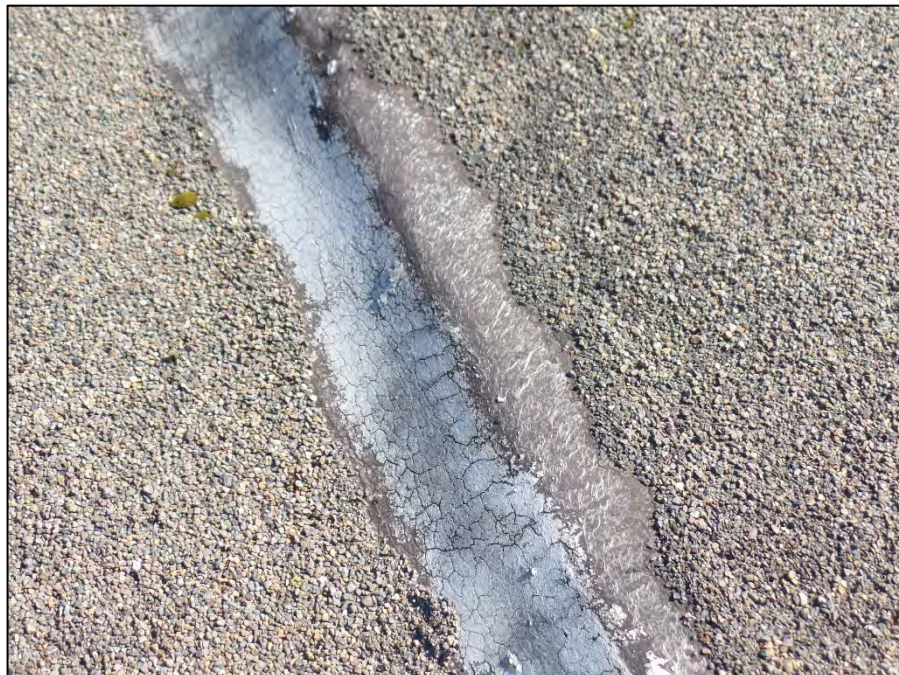
JWE. 1.06 – View of fiberglass exposed in membrane at large roof top unit at the northwest section of the roof.
