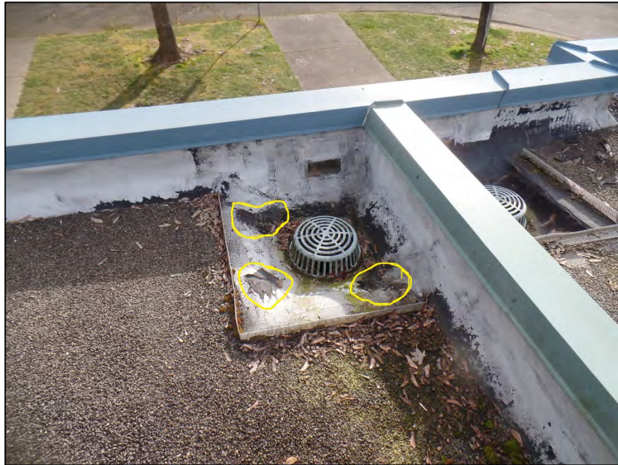
EE. 1.03 – View of typical roof drain & overflow scupper with previous repairs starting to fail.
