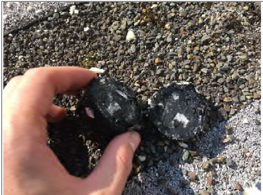
Figure C.12 Moisture identified between walk pad and roofing membrane, outside of roofing system.
