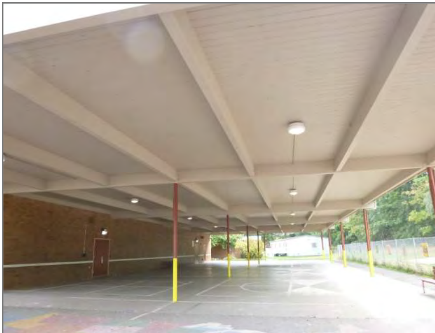
Figure A.10 Electrical conduit and light fixtures at underside of canopy Roof C.
