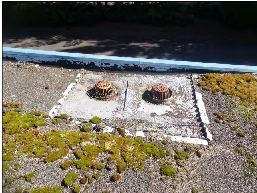
ME. 1.03 – View of typical roof drain and overflow drain with evidence ponding water and moss build-up at the east section of the roof.
