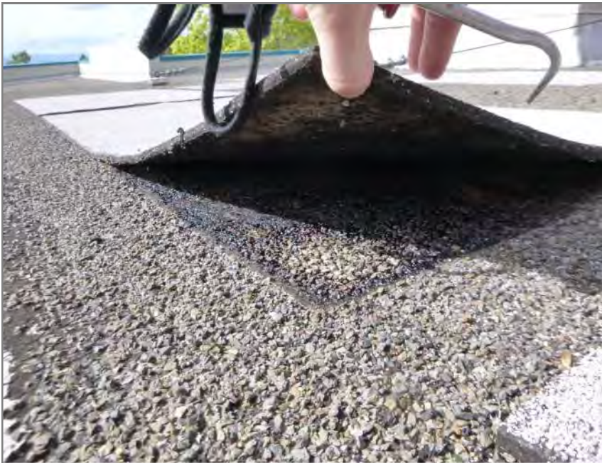
Figure A.9 Moisture trapped between walk pad and roof membrane.
