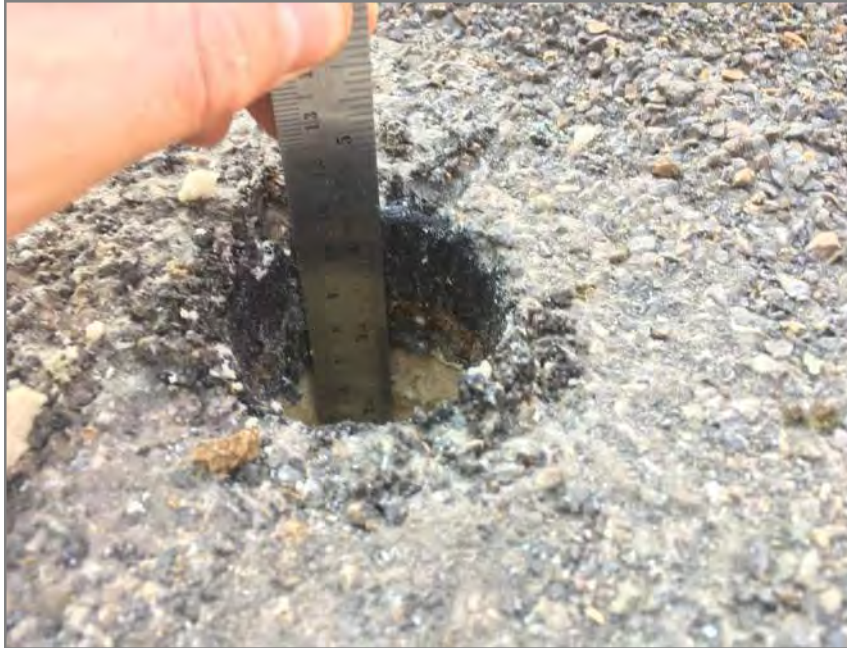
Figure C.7 Roof assembly at rooftop unit pad. 1" BUR membrane 1/2" fiberboard 2-1/2" polyiso insulation Concrete deck
