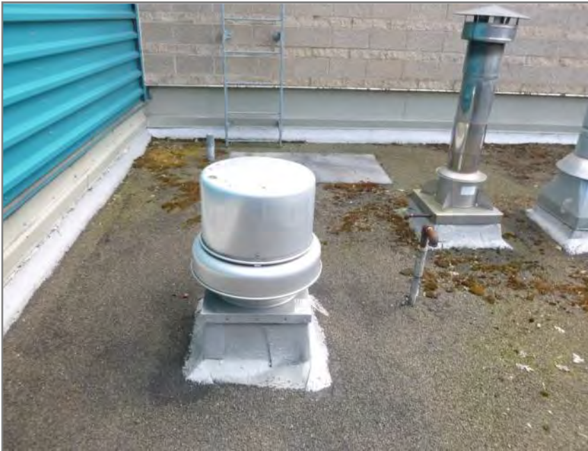
Figure A.13 Moss growth near vent penetrations at Roof D.
