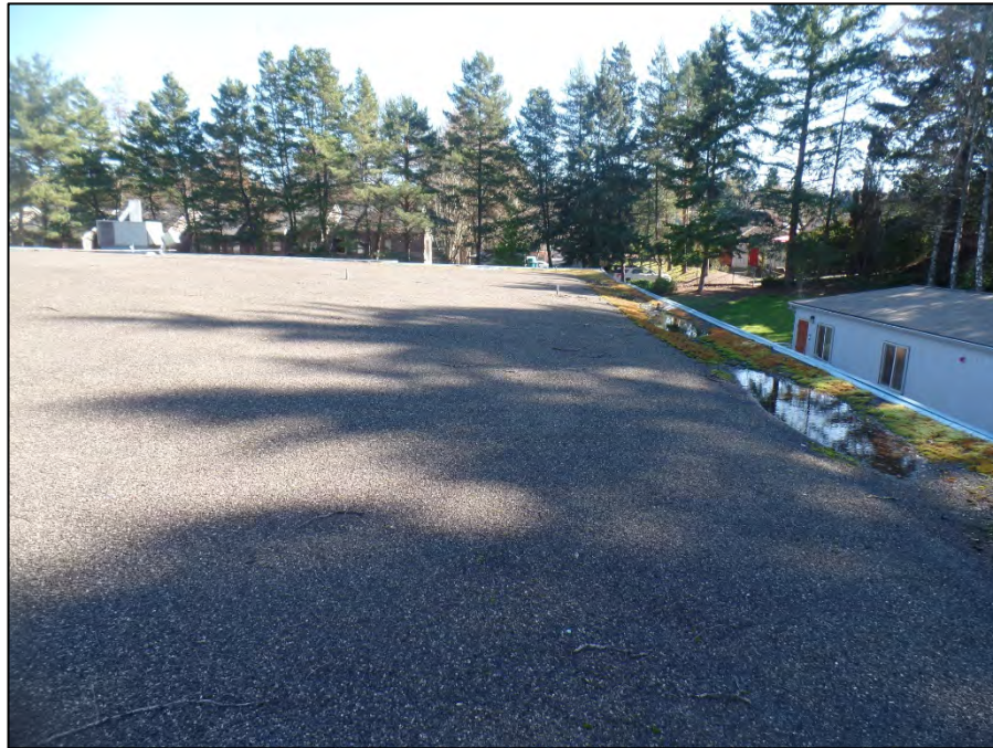
ME. 1.02 – View to east at southwest section of the roof with ponding water and moss build-up.
