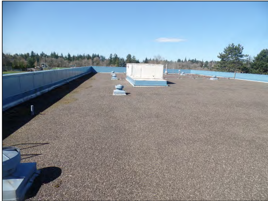
ME. 1.06 – View to west with ponding water and moss build-up along south section of roof.
