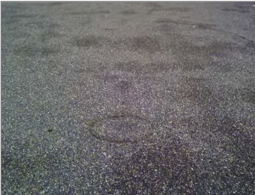
Figure A.12 Example of blister/air bubble (circled) at Roof D
