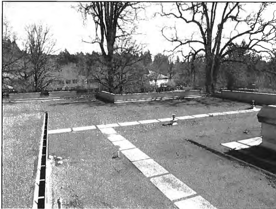
JWE. 1.07– View of moss and organic debris on roof at the southeast section of roof area.
