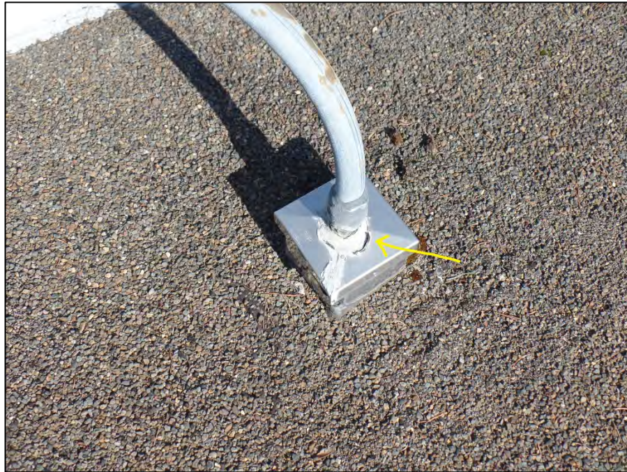
EHE. 1.04 – View of void in the cap of penetration flashing at northeast section of roof.
