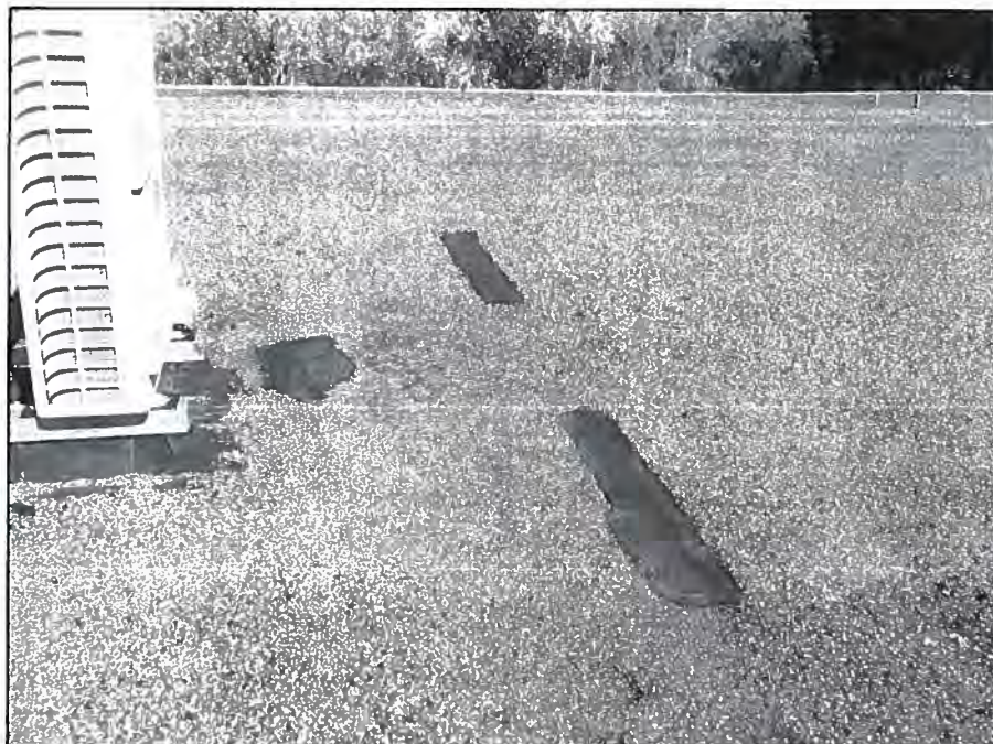
ME. 1.05 – View of typical repairs at the east section of the roof.
