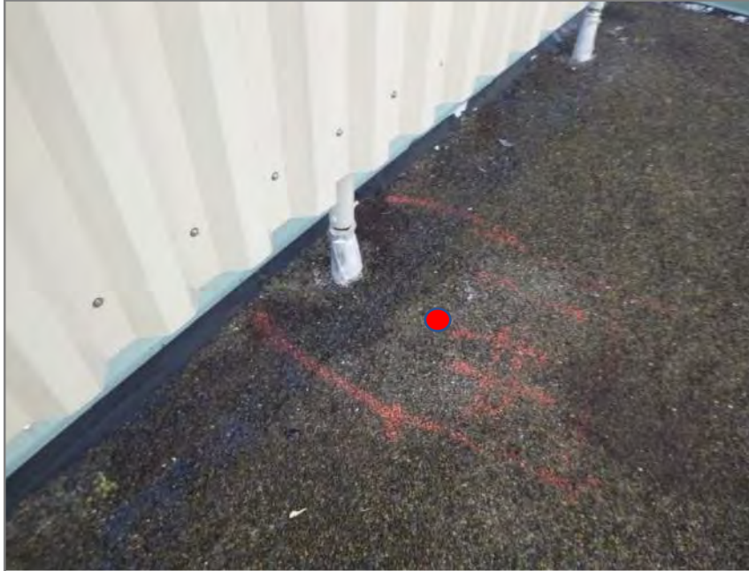
Figure D.1 Core #1 within moisture location #1.
