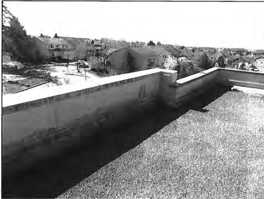
JWE. 1.03– View of typical wall metal and coping flashing at the southwest section of roof, area has had previous leaks.
