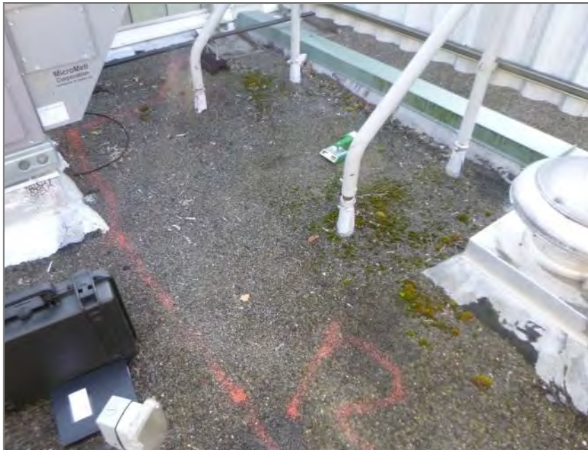
Figure D.24 Electric impedance reading indicates high moisture content within roof assembly at location of core #6 within moisture location #12.
