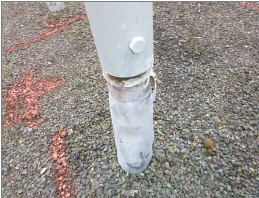
Figure A.6 Thin/failed sealant at mechanical screen support at area #7
