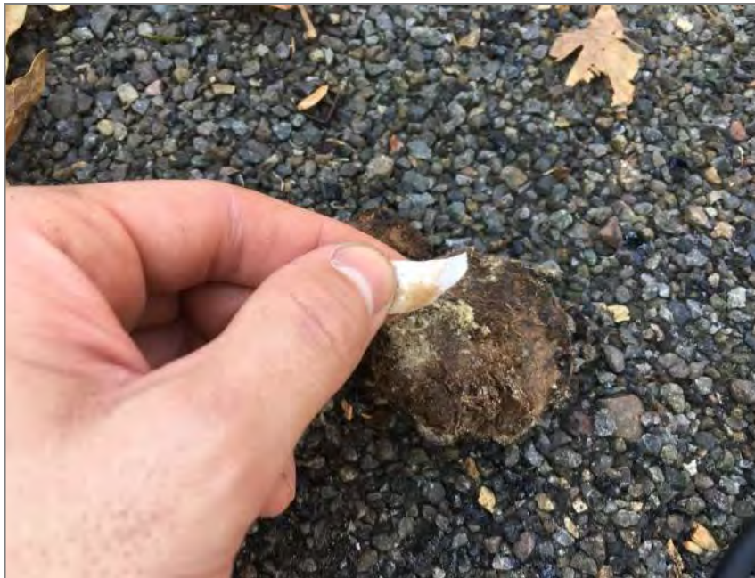
Figure C.16 Fiberboard is wet and deterioration is present.
