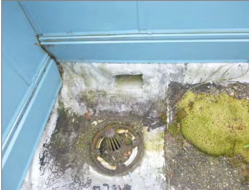
Figure A.9 Typical drain and scupper at Roof D.
