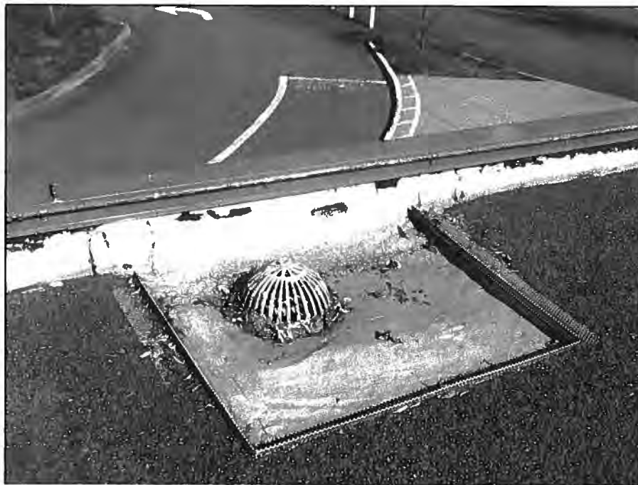
HE. 1.05 – View of typical roof drain and overflow scupper at the northwest section of the roof.
