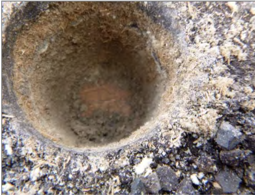
Figure D.4 Insulation and sheathing are dry.
