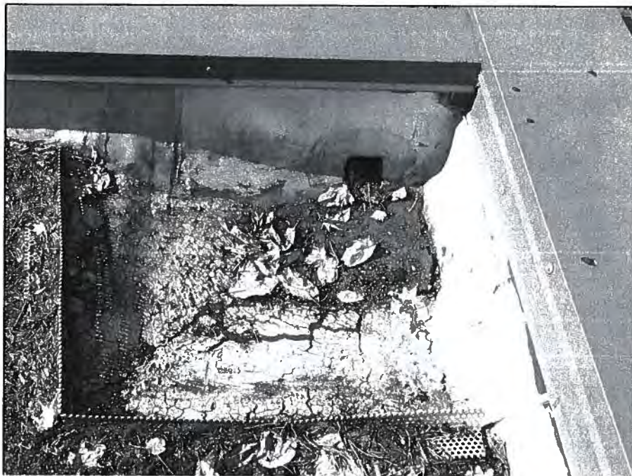
EHE. 1.05 – View of typical roof drain scupper with splits and coating deterioration.
