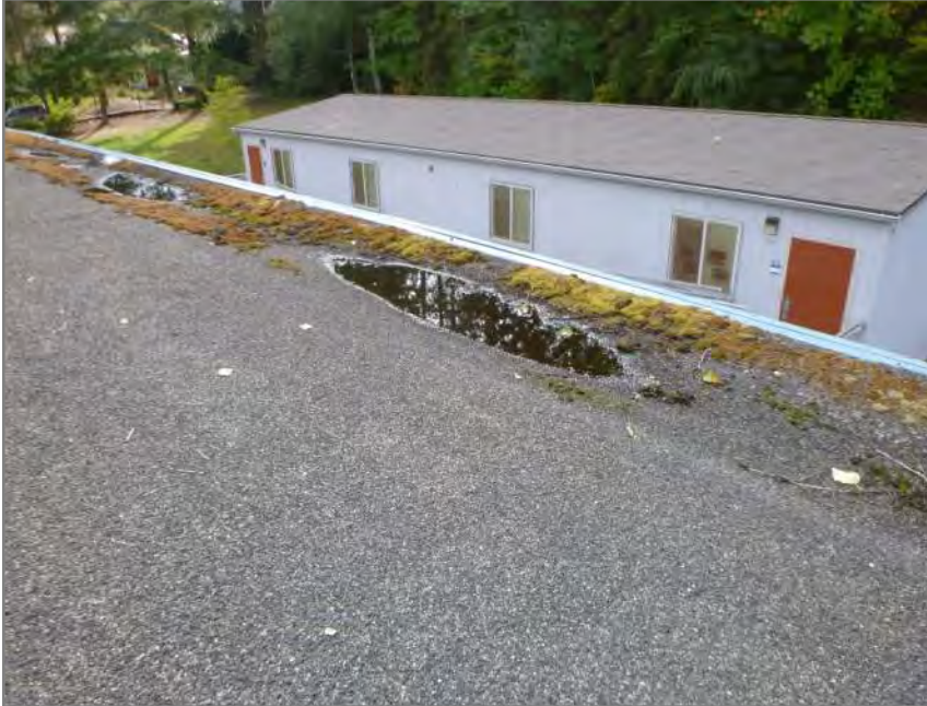
Figure A.11 Standing water along south perimeter at Roof A.
