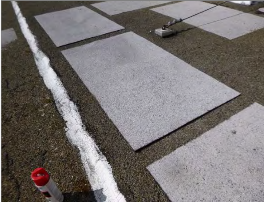
Figure A.8 Typical walk pad on roof surface.
