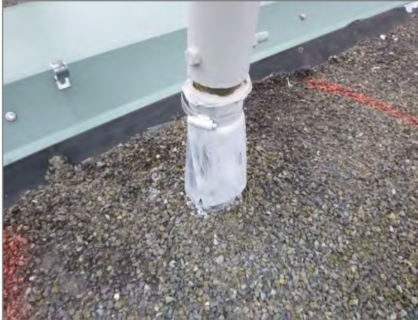
Figure A.5 Typical mechanical screen support with painted lead skirt flashing.
