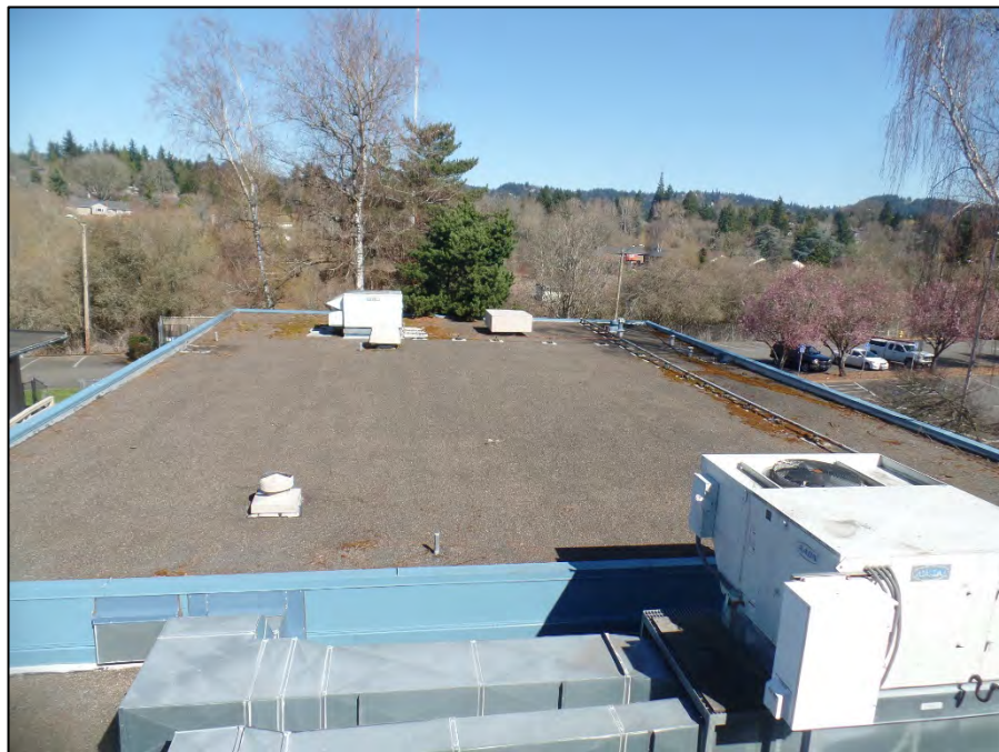
ME. 1.07 – View to the north of northwest roof with evidence of moss build-up.
