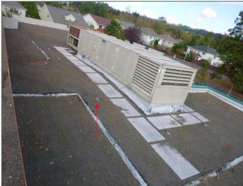
Figure A.15 Air handling unit with seismic anchor cables.
