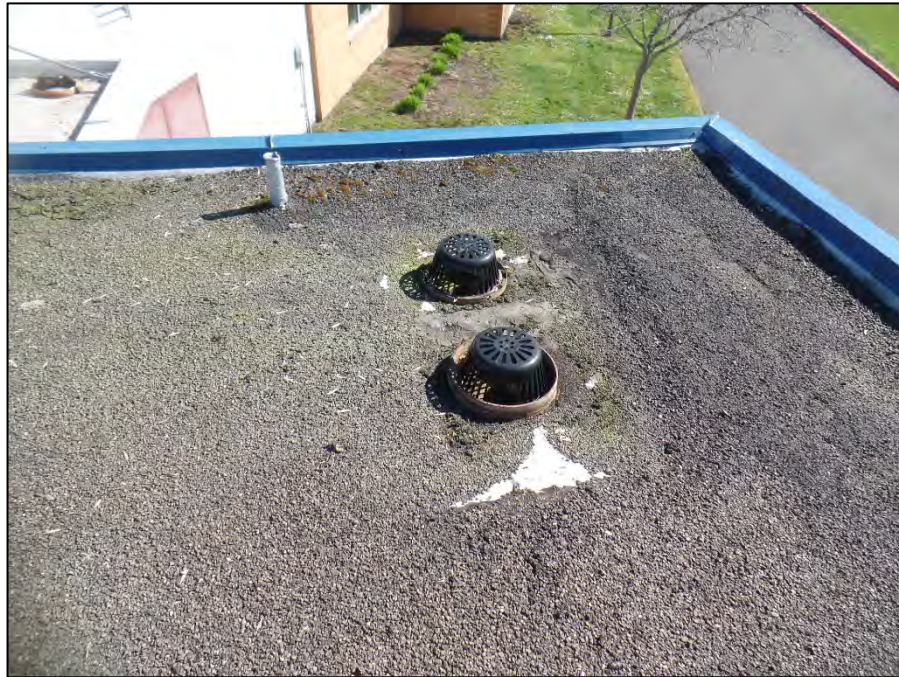
HE. 1.04 – View of typical roof drain and overflow drain at the east section of the roof.
