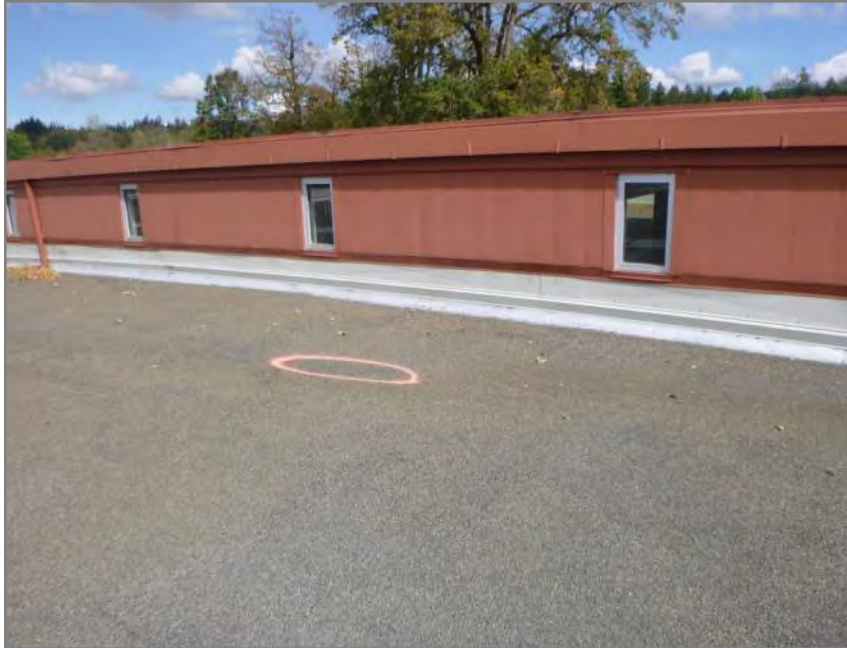
Figure A.14 Air bubble/blister identified along cricket edge at Roof A.
