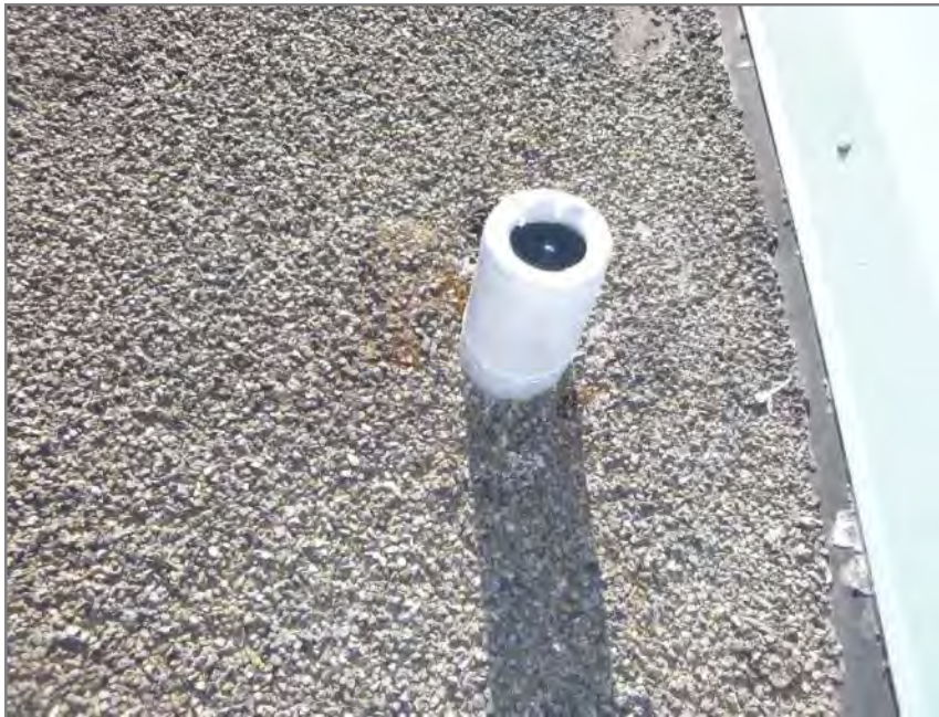
Figure A.4 Typical vent penetration.
