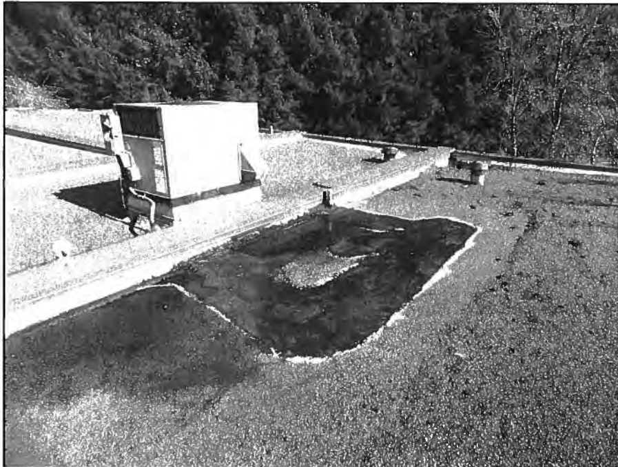
EHE. 1.03 – View of repair at current interior leakage area at northeast section of the roof.
