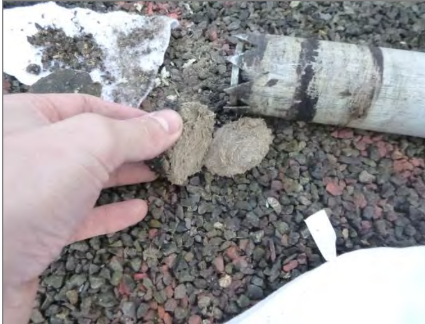
Figure D.9 Fiberboard deterioration noted.
