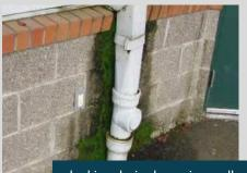
leaking drain damaging wall
