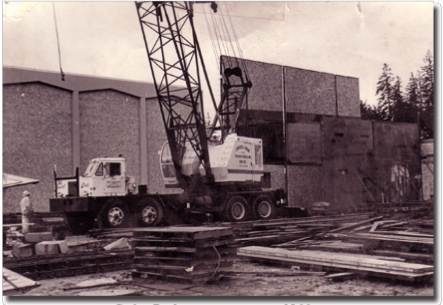
Cedar Park construction site, 1966.
